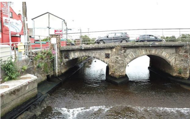
South Embankment and Span No1
