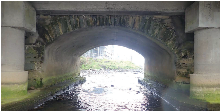
Mortar erosion from upstream face of masonry requires re-pointing
