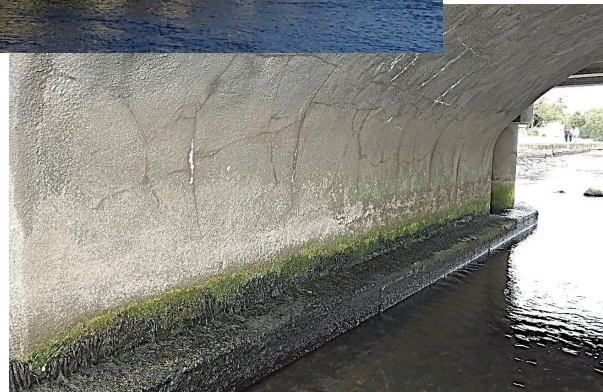
Note lime leaching to some arches in the form of white Calcium carbonate deposits. This signifies loss of fabric from deep within the arch masonry and indicates water penetration through the deck.
