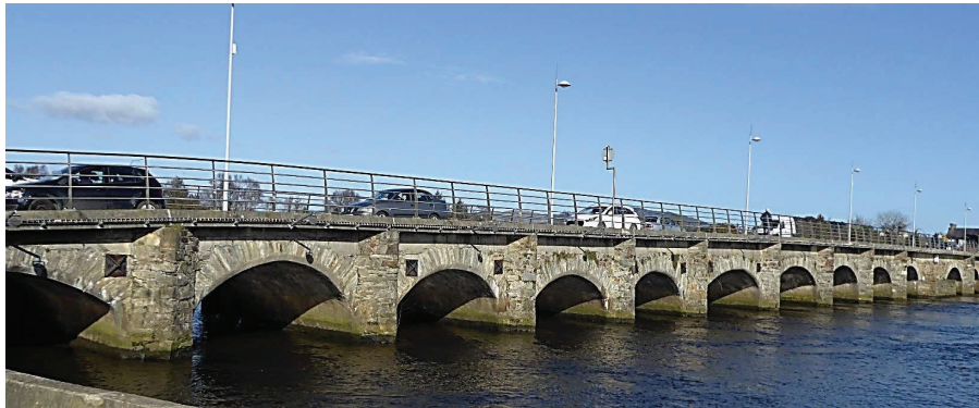
Note lime leaching to some arches in the form of white Calcium carbonate deposits. This signifies loss of fabric from deep within the arch masonry and indicates water penetration through the deck.
