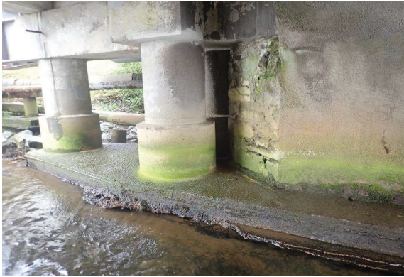
North Bank - west side - view from arch 18
