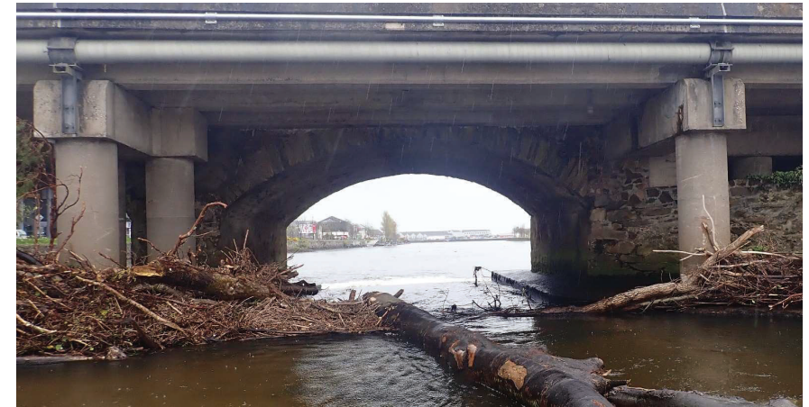
Attrition from floating debris is damaging stonework. Tree trunks etc catch between newer piers and historic masonry. New works should include measures to prevent such The proposed new debris trap upstream should alleviate this issue
