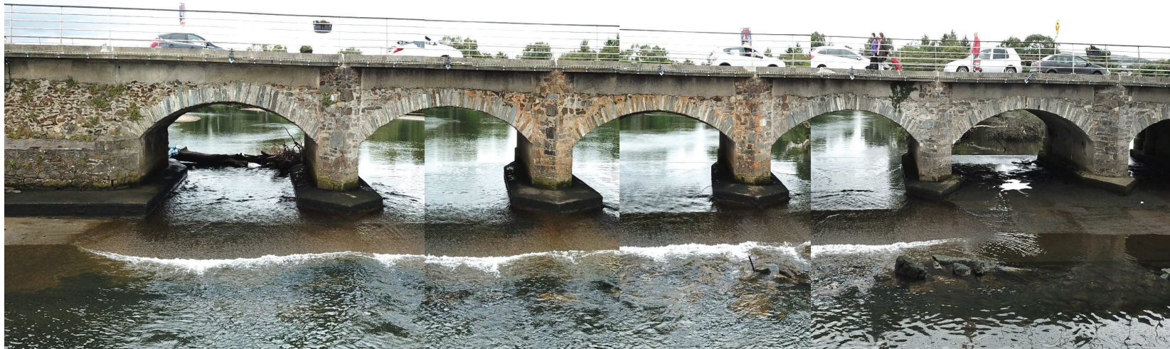
Attrition from floating debris is damaging stonework. Tree trunks etc catch between newer piers and historic masonry. New works should include measures to prevent such The proposed new debris trap upstream should alleviate this issue
